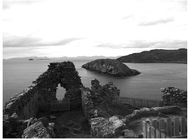
Duntulm Castle stands ruined on the north coast of the Isle of Skye in Scotland near the hamlet of Duntulm.
